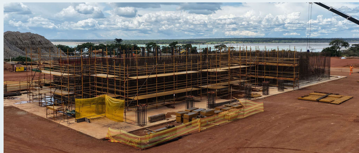
Mill building civil works, Lumwana expansion
